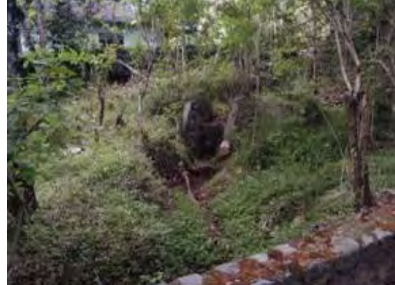
Gully plug constructed under IBRD project in Keduang watershed
