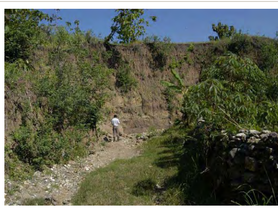
River bank erosion and protection in Giriwoyo, Alang watershed
