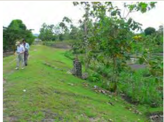
Maintaining of a small storage reservoir in Giriwoyo, Alang watershed
