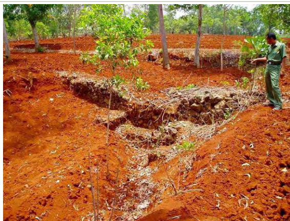
Broken gully plug in Keduang watershed
