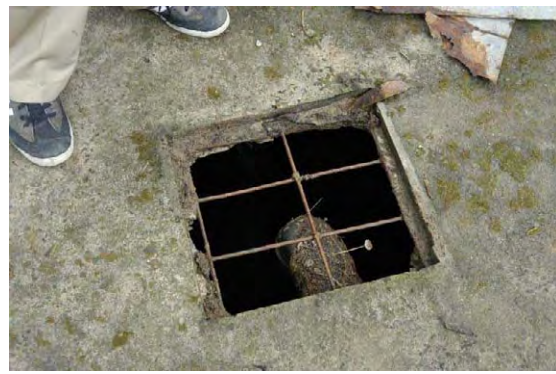
Water tank (about 20m 3 ) in the settlement area for storing rainfall constructed by IBRD project in Keduang watershed
