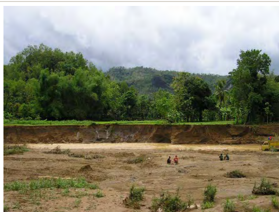
River bank erosion in Solo River
