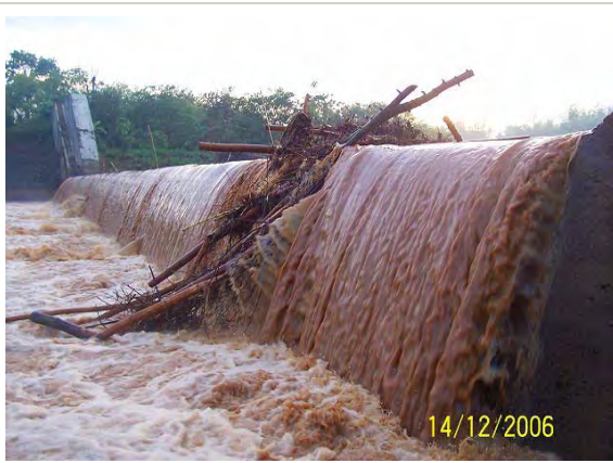
Garbage overflowing on check dam in Keduang River on December 14, 2006
