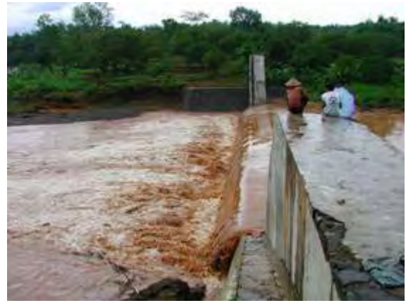
Check dam in Keduang watershed
