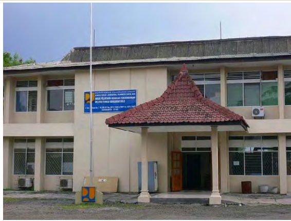
PBS (Bengawan Solo River Basin Development Office) Office, Surakarta
