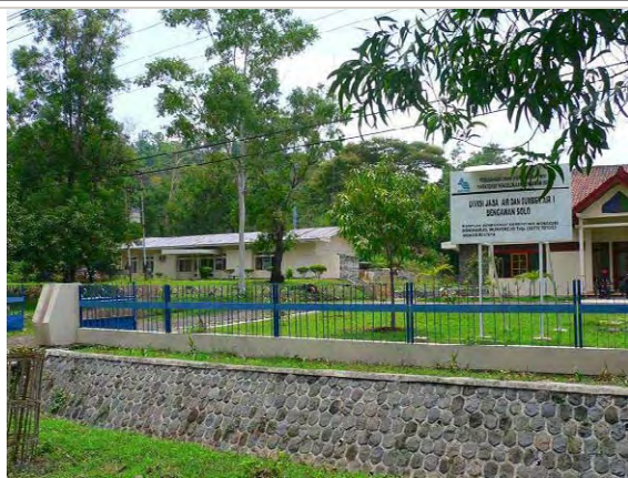
PJTI Bengawan Solo Wonogiri Dam Office, Kabupaten Wonogiri
