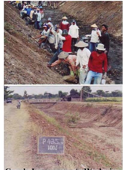
Canal Improvement Work in 2004 (Source: Balai PSDA)
