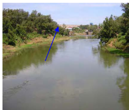
D/S of the Wonogiri Dam
