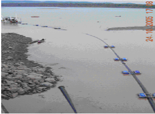
Photo 2.4.1 Barge and Discharge Pipe
