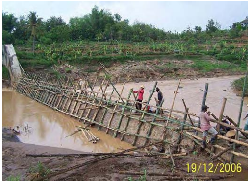
Installation of garbage trap by bamboos
