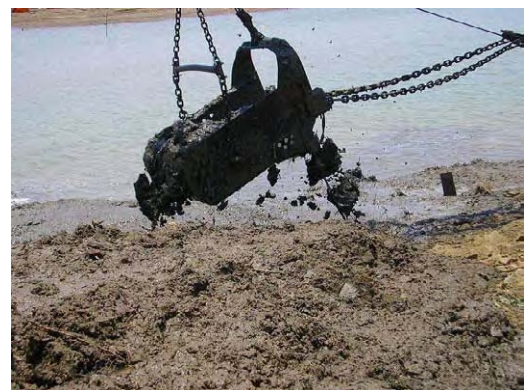
Excavation of sediment deposits at the intake by a dragline in October 2006
