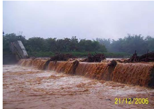
Broken garbage trap by flood
