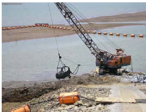
Excavation of sediment deposits at the intake by a dragline in October 2006
