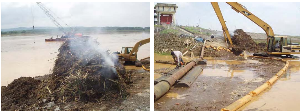
Photo: Debris removal in January, 2004
