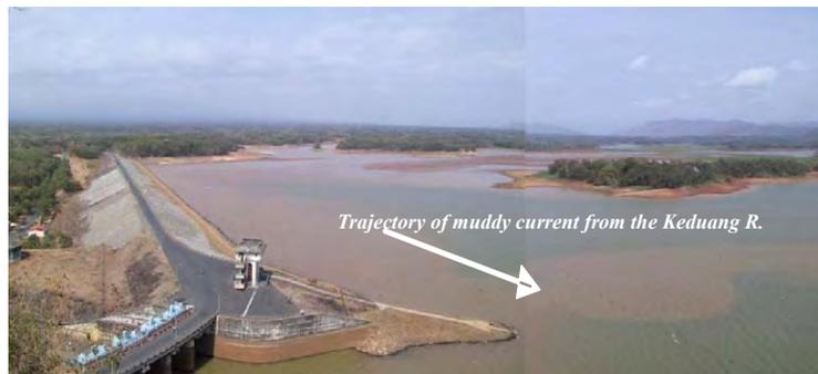
**Photo Trajectory of Flood Flow (Muddy Current) in the Reservoir**
