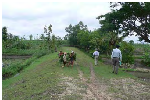
Check Dam in Alang Area
