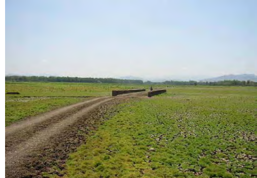
Sediment Deposits at the old bridge on the Reservoir Arm of Alang River
