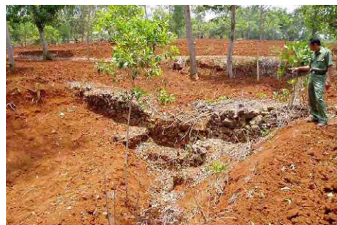
Small Gully Plug in Keduang Area
