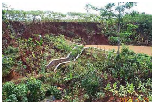
Large Gully Plug in Keduang Area
