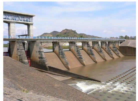
Colo Intake Weir
