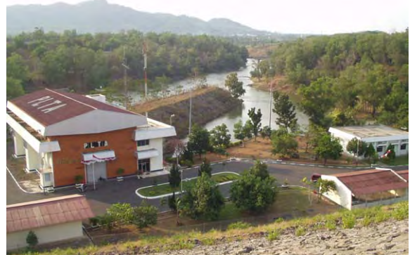
Wonogiri Power Station
