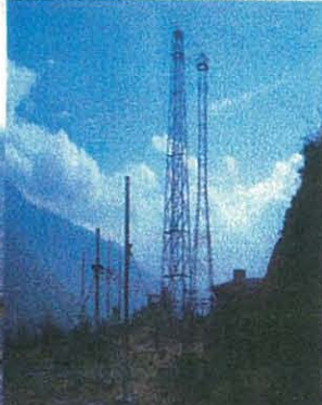
Installation of New 100 KW SW Transposer at Sanggyag
