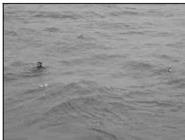
Photo J. 8.2.12: Fixing work of apparatus by divers
