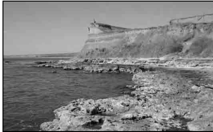
Photo D.1.1: Eroded limestone at the foot of the cliff at the south of Hotel Horum at Southern Costinești
