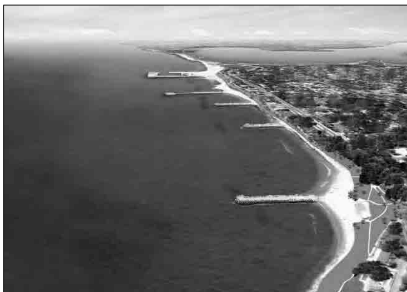
Fig. 4.1.1: Bird’s-eye view of the beach before project implementation at Eforie Nord
