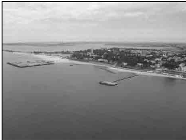
Photo-25 Aerial View of Shore Protection Facilities in Eforie Nord
