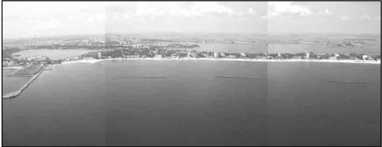
Photo-1 Aerial View of Project Site for Mamaia South
