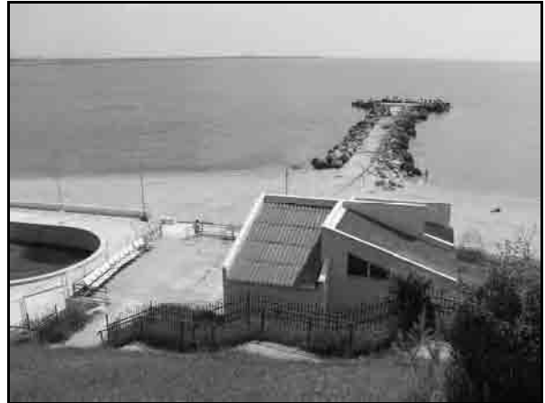
Photo-24 Shore Protection Facility in Agiea
