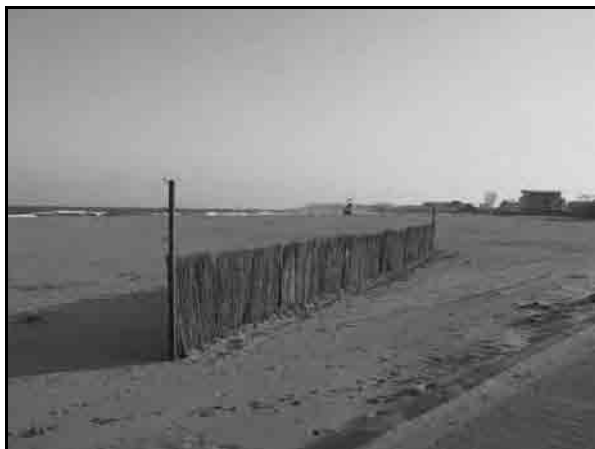
Photo-16 Wind Blown Sand Fence in Mamaia South
