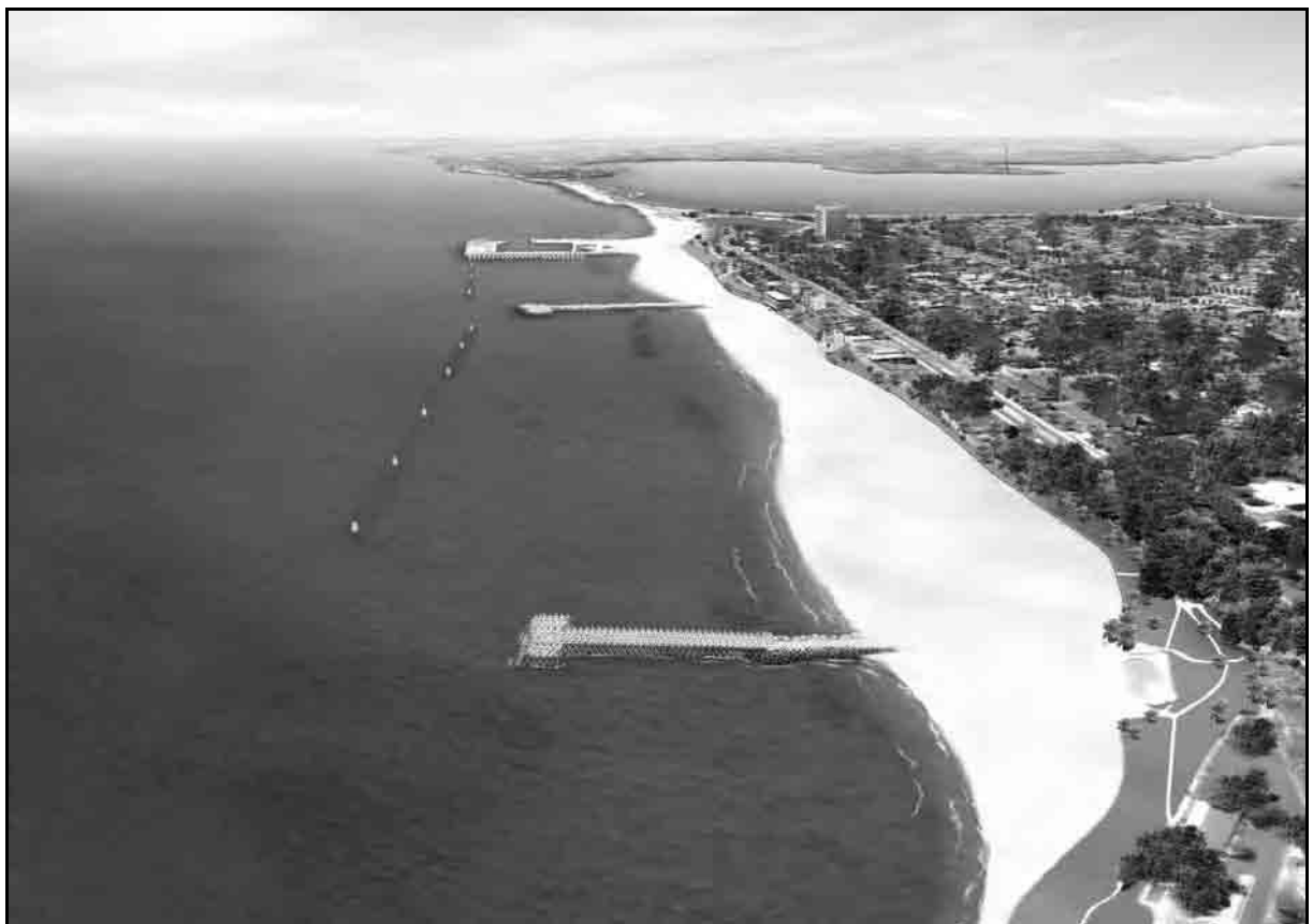
Eforie Nord before Project Implementation
