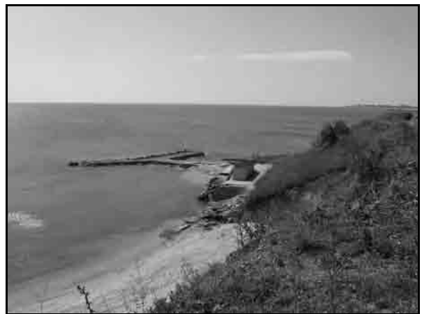
Photo-22 Shore Protection Facility in Agigea
