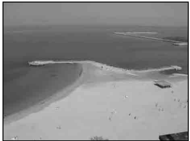
Photo-9 Shore Protection Facility in Mamaia South
