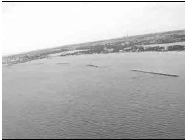
Photo-6 Offshore Breakwaters in Mamaia South
