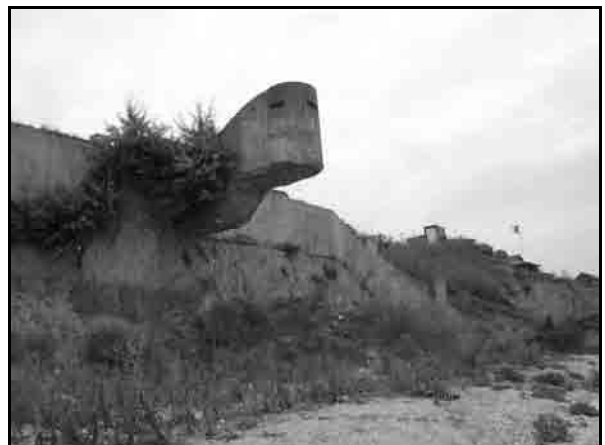
Photo-48 Cliff Scouring Condition in Schitu
