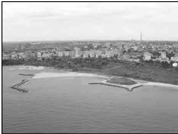
Photo-19 Shore Protection Facilities in Tomis South
