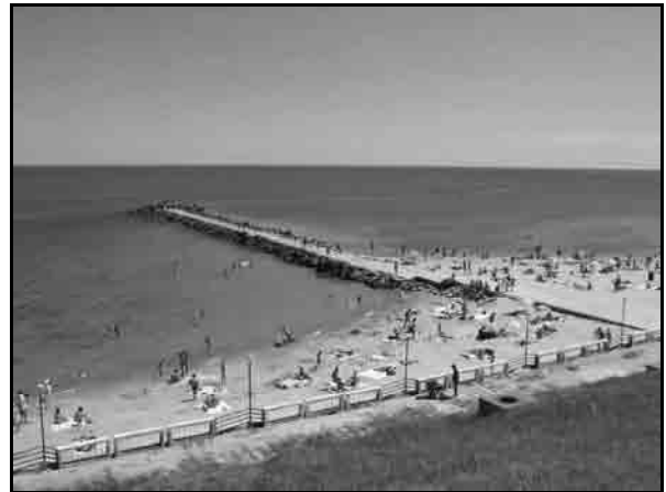
Photo-40 Shore Protection Facility in Eforie Sud
