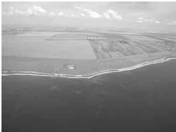
Photo-47 Aerial View of Schitu
