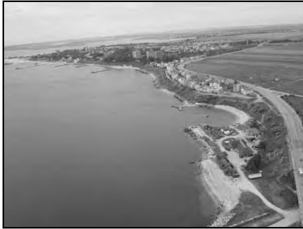
Photo-25 Aerial View of Agigea
