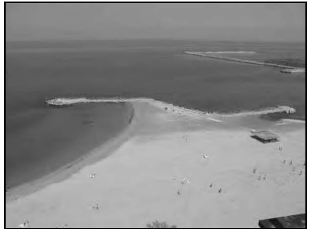
Photo-16 Shore Protection Facility in Mamaia South
