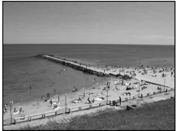
Photo-40 Shore Protection Facility in Eforie Sud
