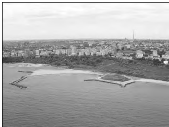
Photo-19 Shore Protection Facilities in Tomis South
