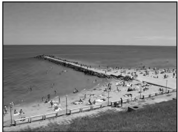
Photo-40 Shore Protection Facility in Eforie Sud
