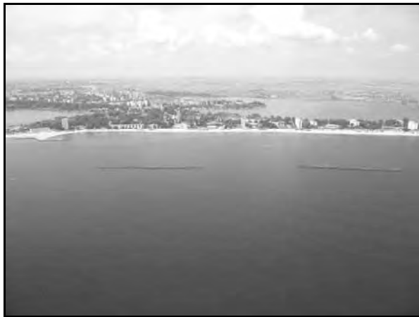
Photo-13 Aerial View of Mamaia South
