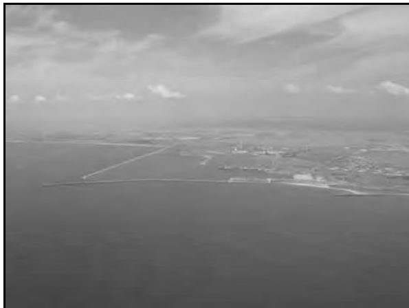
Photo-3 Aerial View of Midia Port
