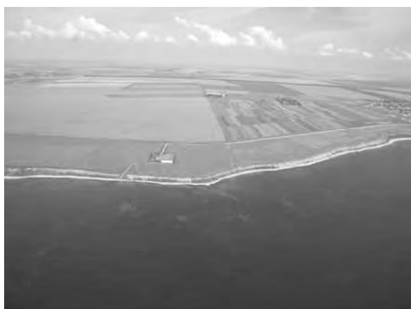
Photo-47 Aerial View of Schitu
