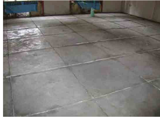
(Phuentsholing HSS) 1階床下地施工
