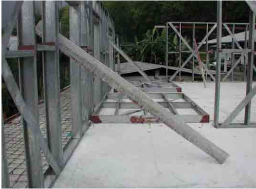
(Phuentsholing LSS) 2階壁骨組み建て方
