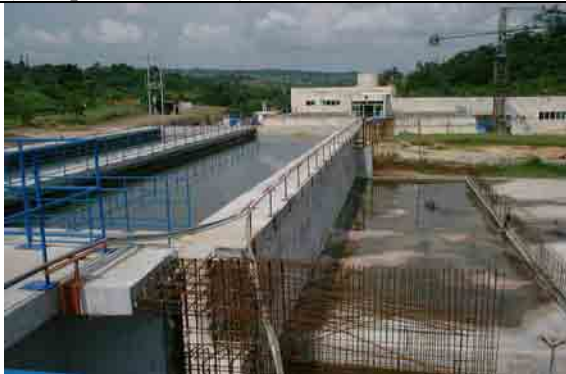
Sedimentation, Filtration and Operation Building
