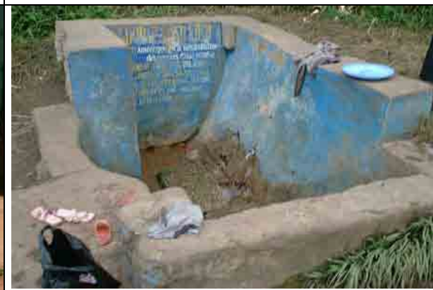
Communal Water Supply Pint at the Kusukusu River
