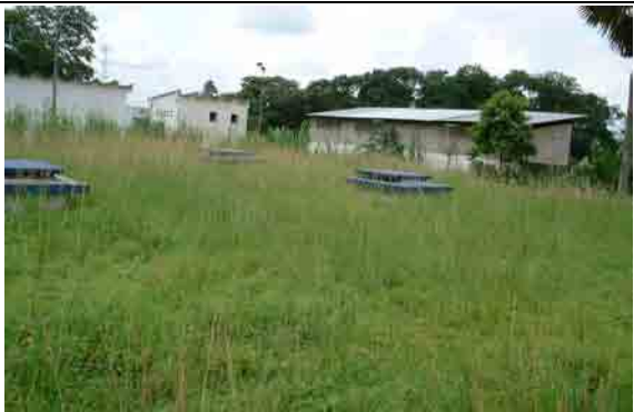
Reservoir and Pump Station
