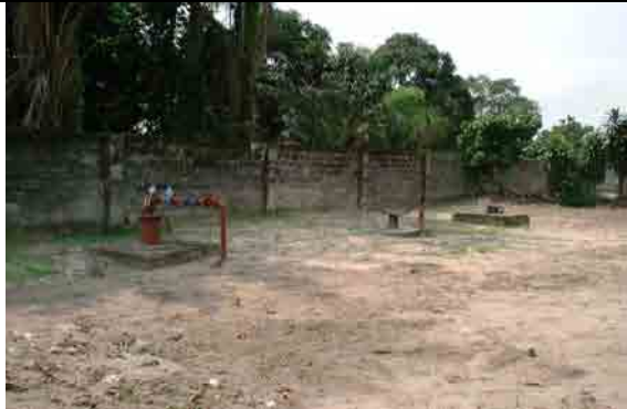
Two Boreholes Yield: 20 m 3 /h/borehole Only one borehole is operating
