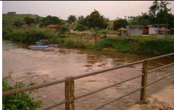
Site for WTP
