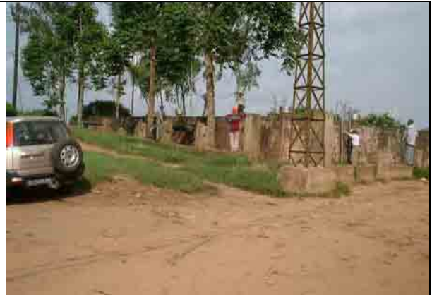
Main Reservoir (1,200 m 3 )
