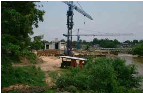
Intake facilities Under construction with the assistance of WB (Mod.3)
