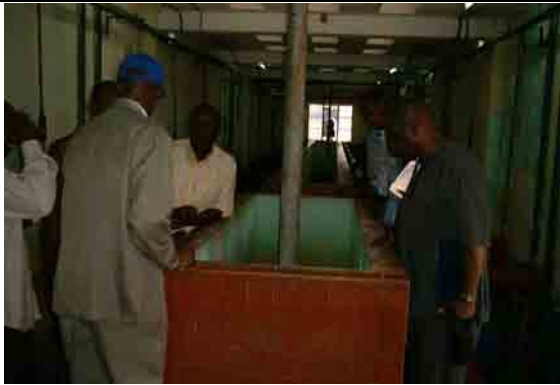
Mixing Tank for Coagulation
