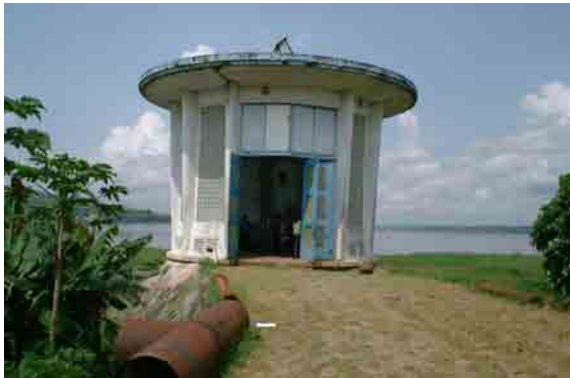
Intake Pump Station
