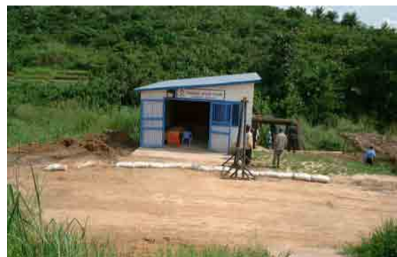
Temporary intake pump station
