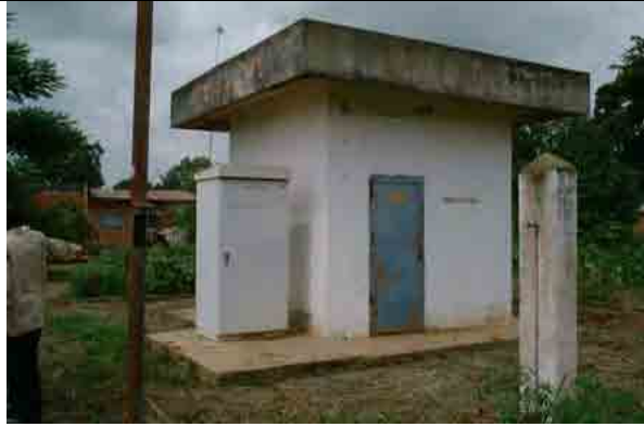
Well No. 7: Dry up after 2 months
