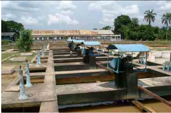
Overview Coagulation, Sedimentation and Filtration
