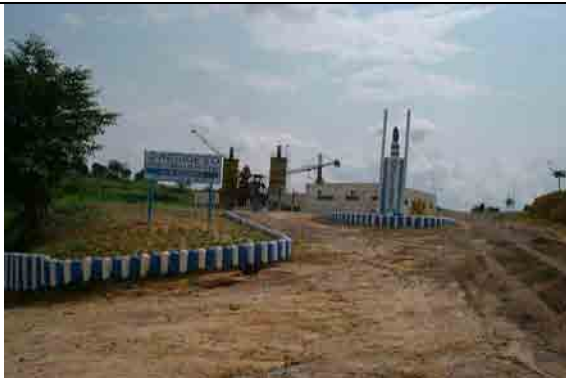
Overview Under construction by REGIDESO (Completed in 2008)
