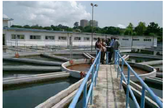
Sedimentation Tank
