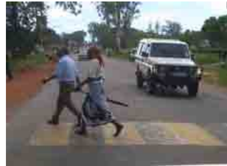
Photo 2.4 Crossing based on Malawian standards. The narrow width of 2m creates low visibility for drivers.
