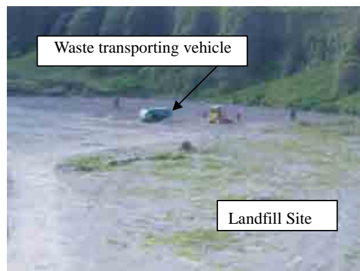
Pokhara Sanitary Landfill Site at the Seti and Phurse River Confluence
