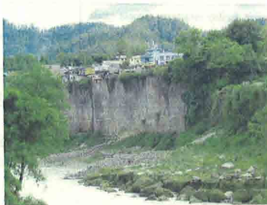
Erosion-prone area of Bhimad Bazaar
