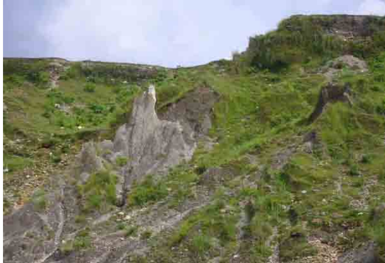
Plate 7: Intense gully erosion on the soil slide and river terrace on the right bank of Jyagdi Khola
