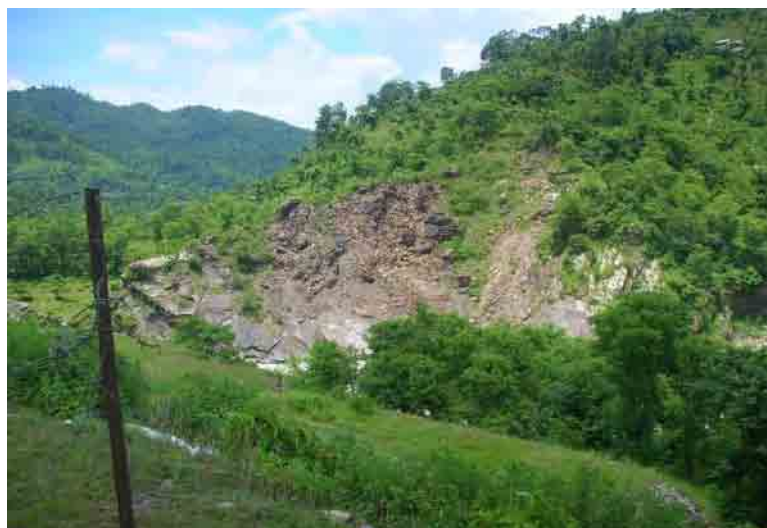
Plate 5: Rockslide on the left bank of The Seti River near Bhimad Bazaar
