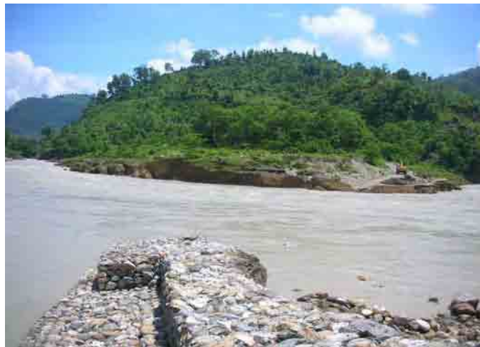
Plate 3: River training works to protect the bank cutting
