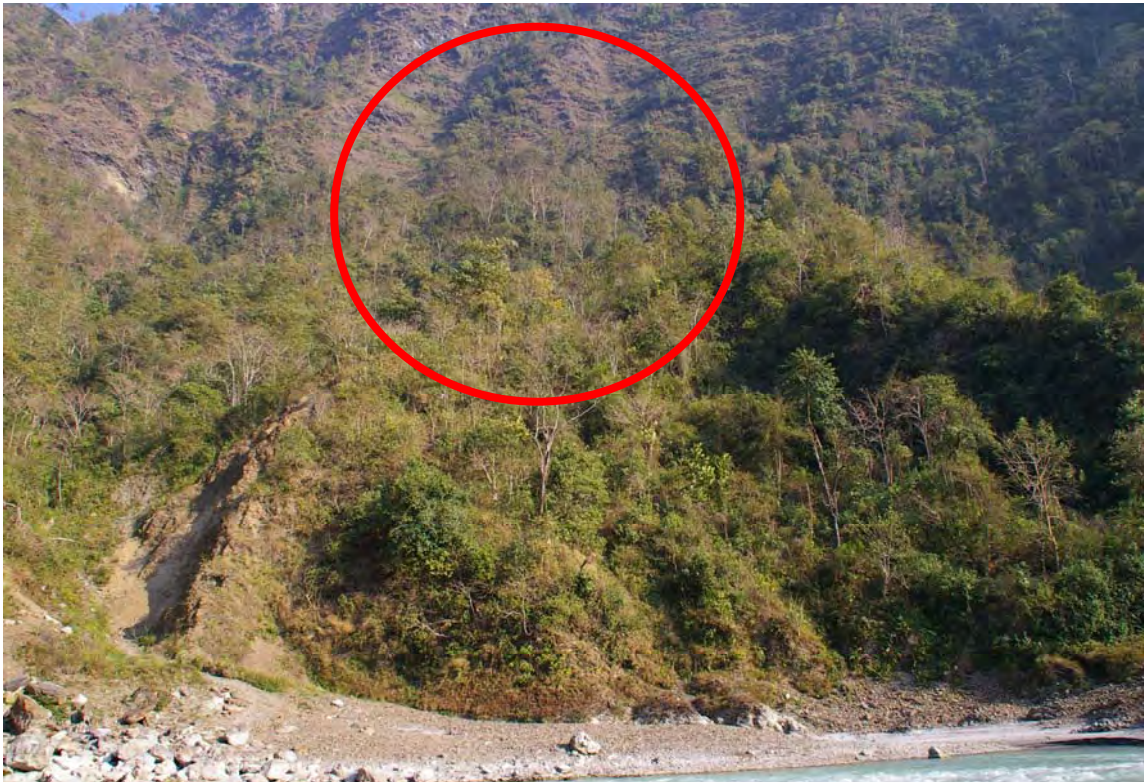
View of Intake
