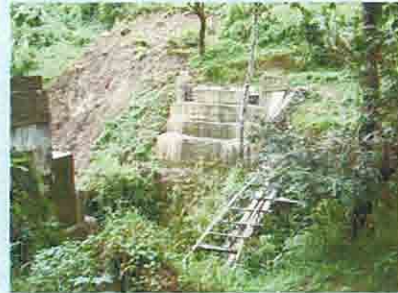
Malucsad site 80m from road end to Power house site
