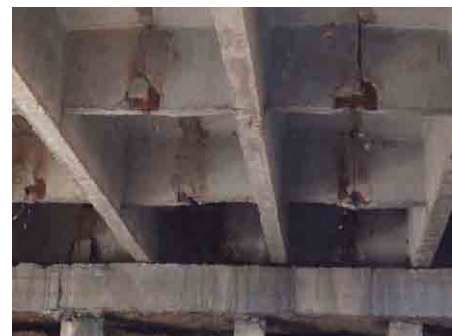
Discontinuous Cross Girder
