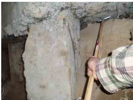
Inspection by a Test hammer
