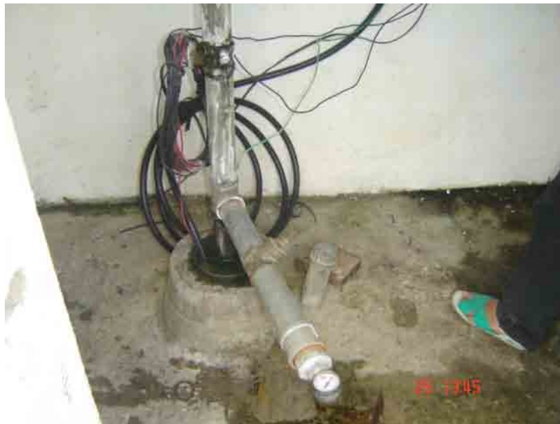
Figure 6. The deep well as source of water for Kiotoy Water System.
