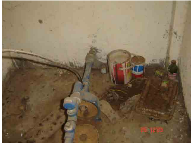
Figure 4. The dismantled centrifugal pump and motor at the pump station.
