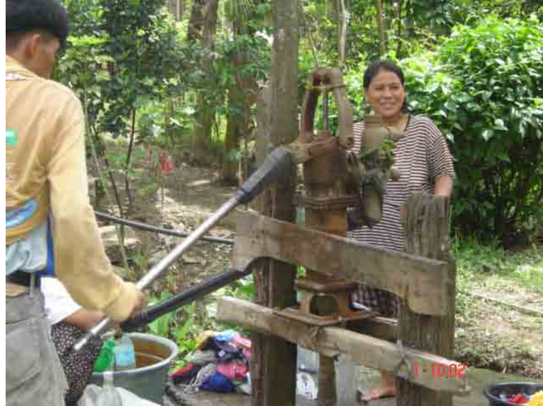
Figure 2. The jetmatic pump of the Olaycon Water System.
