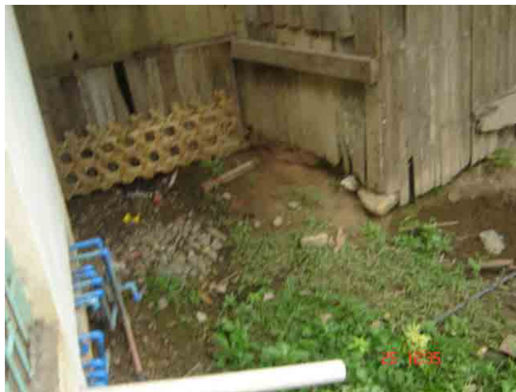
Figure 5. The one- inch pipes distributed to the different households.
