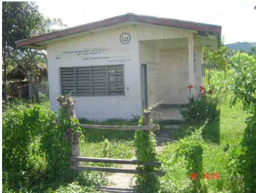
Figure 1. The abandoned office of the system.
