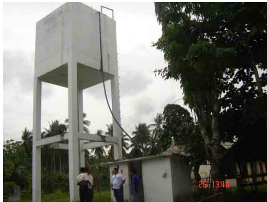
Figure 8. The reservoir is fed by 2 inch PE pipe from the pump house.
