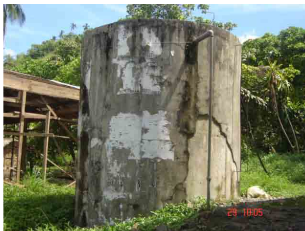
Figure 3. The reservoir at Barangay Mayo.
