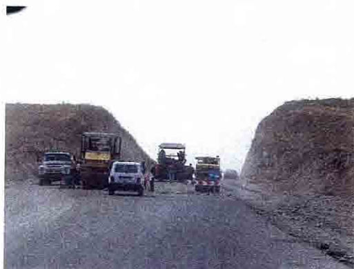
As 敷設作業
