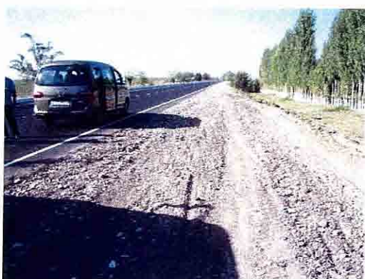
Tashkent-Jizzax間拡幅工事
