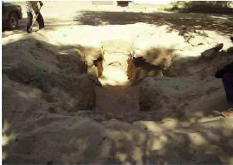
Back fill work for old pit B
