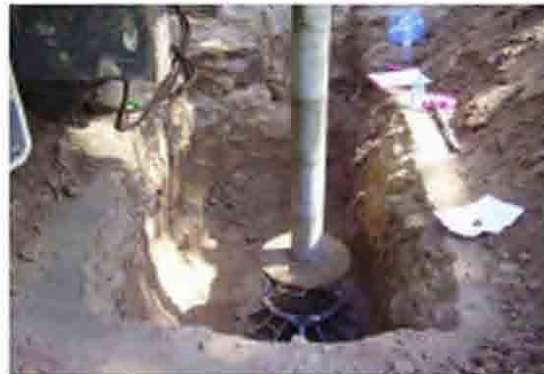
Plat load test of new pit B In progress
