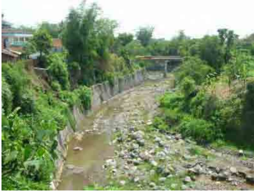
③護岸工と堰堤
