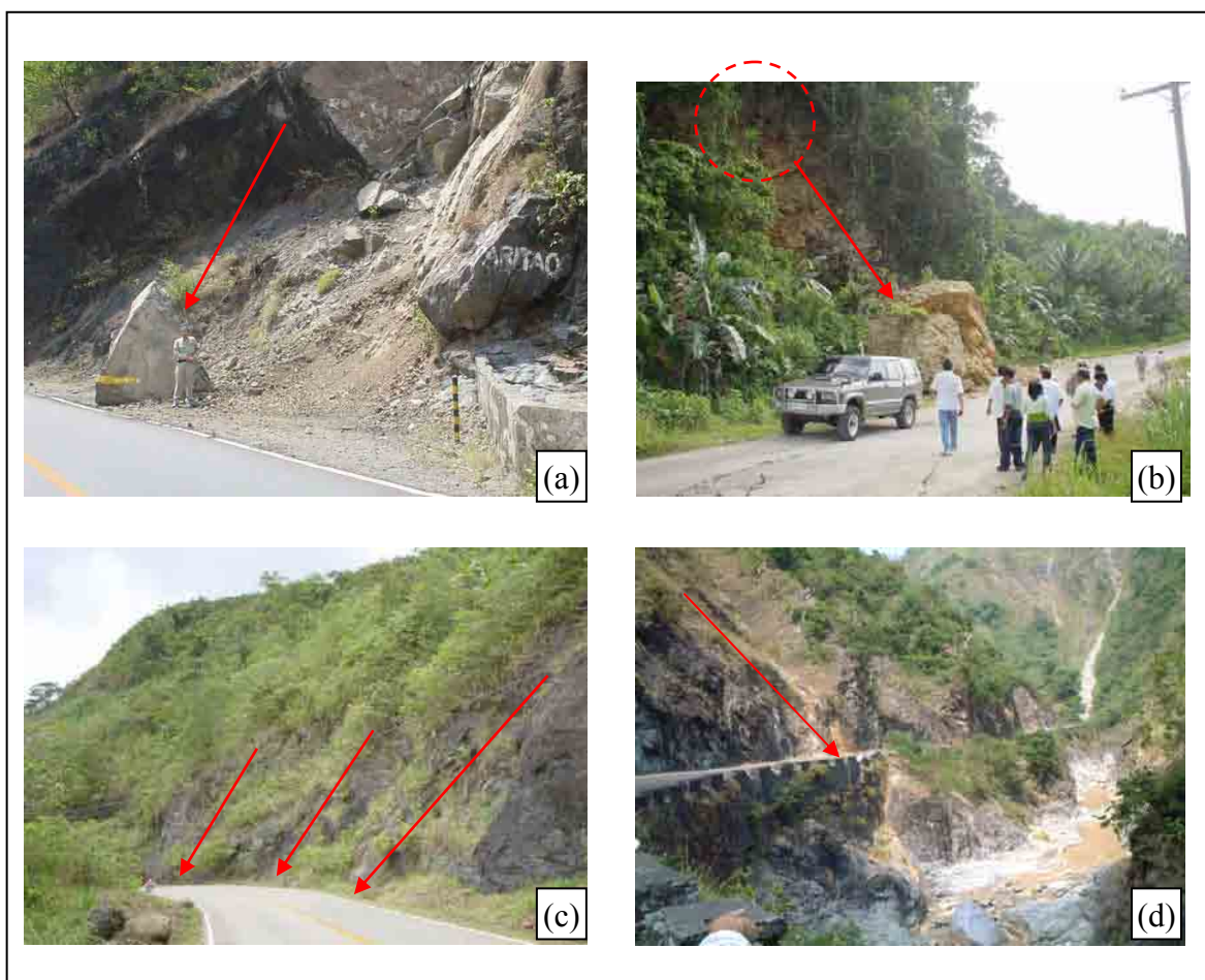
Figure 2.9 Rock Slope Collapses Occurring along the National Highways
