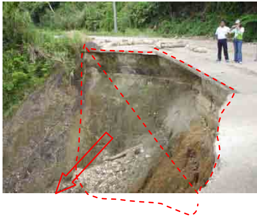
Figure A2.15 Road Slip (RS) Slip of roadway and valley side slope along Wright-Taft Road (km 858+250)
