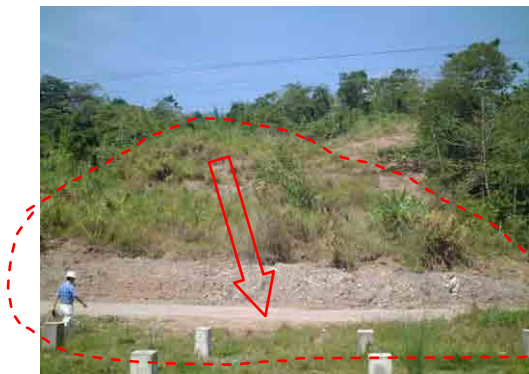
Figure A2.10 Landslide (LS) along Banaue-Lagawe Road (km 301+200)
