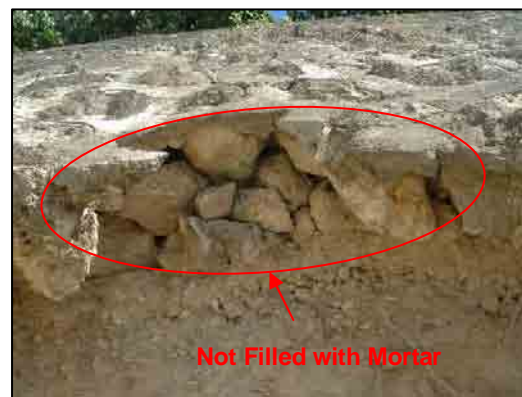
(b) Inside of Grouted Riprap Wall
