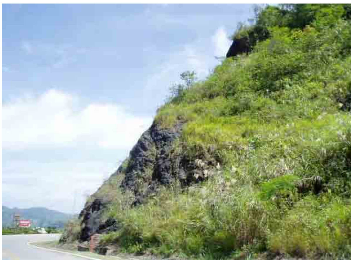
Figure 5.23 General View of Example DIS Slope for Rock Slope Collapse
