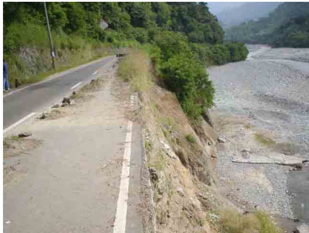
Figure 5.41 General View of Example DIS Slope for River Erosion
