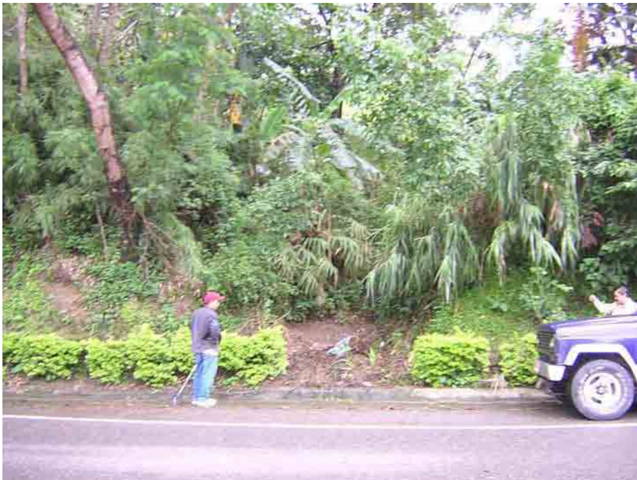
Figure 5.35 General View of Example DIS Slope for Debris Flow
