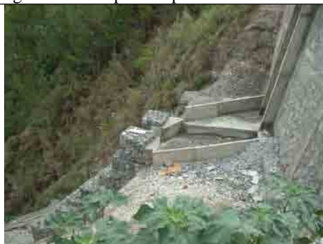
Surface drainage to protect against road slip
