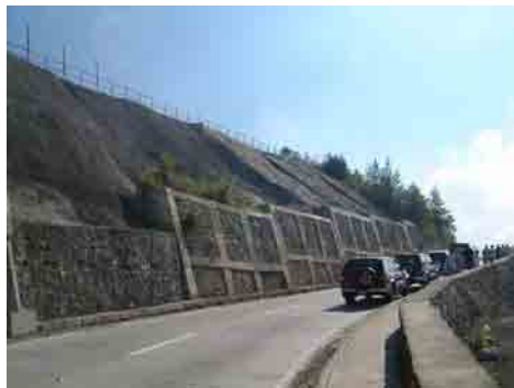
Concrete crib masonry wall to protect against soil slope collapse
