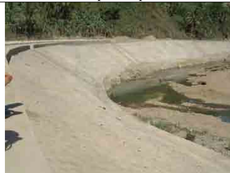
Revetment to protect against river erosion
