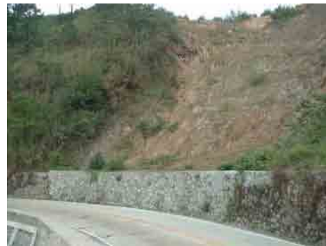
Cutting and masonry wall to protect against soil collapse
