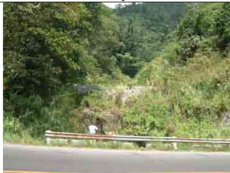
Masonry sabo dam to protect against debris flow
