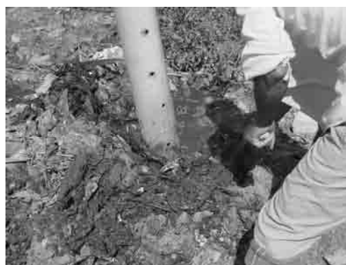
Photo 1.4 Condition of Gas Ventilation Facility
