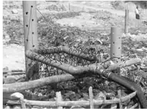
Photo 3.12 Leachate Re-circulation Bed
