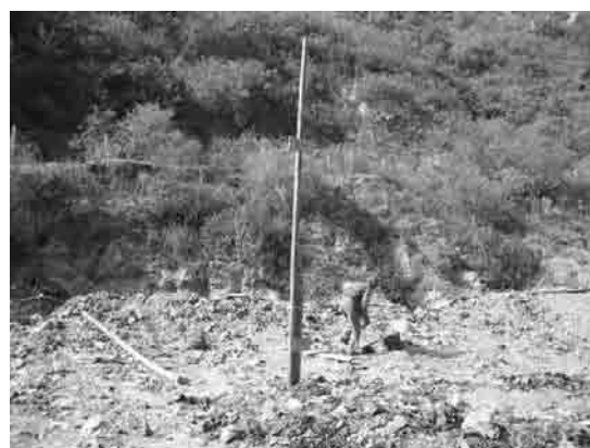
Photo 2.15 Finishing Stake Installed
