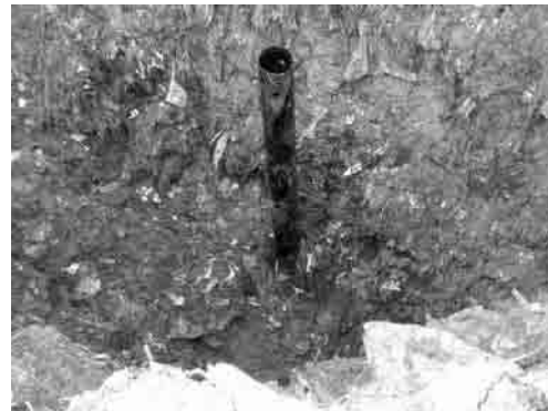
Photo 2.4 Excavation to GL -3.0m
