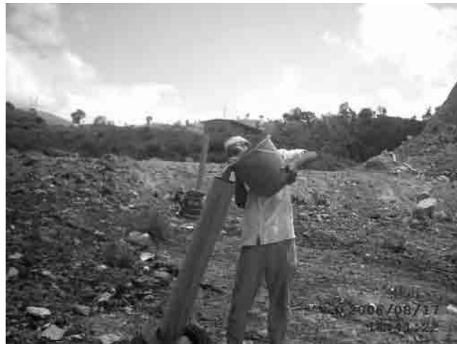
Photo 2 Pouring Colored Water into the Gas Ventilation Pipe
