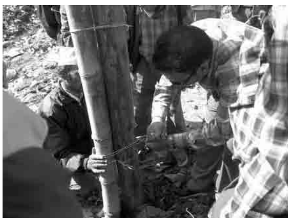
Photo 2.14 Fixing Finishing Stake
