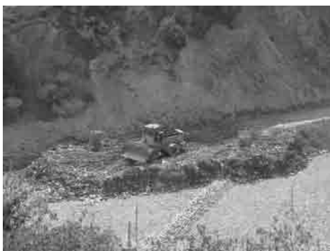
Photo 3.27 Landfill Compaction by Landfill Compactor
