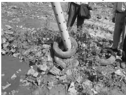
Photo 1.3 Gas Ventilation Facility
