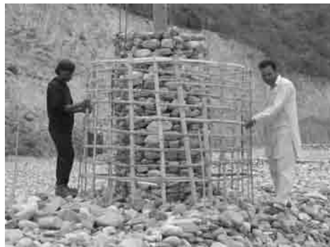
Photo 3.30 Improved Gas Ventilation Facility
