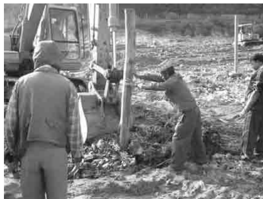
Photo 2.13 Installation of Finishing Stake
