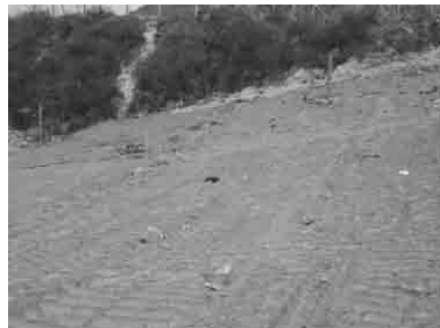
Photo 3.20 Final Soil Cover (No. 2)
