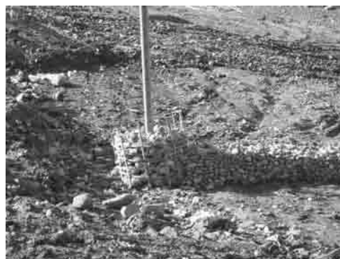
Photo 3.2 Bamboo Gabion
