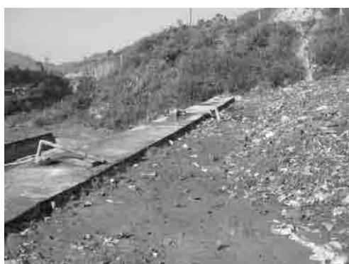
Photo 2.16 Site Requiring Preventive Net
