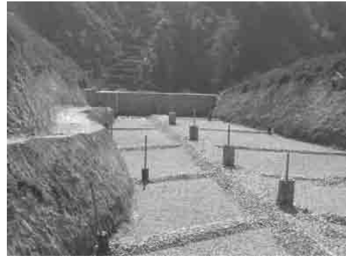
Photo 3.21 On-site Road of Left Bank of Valley 2
