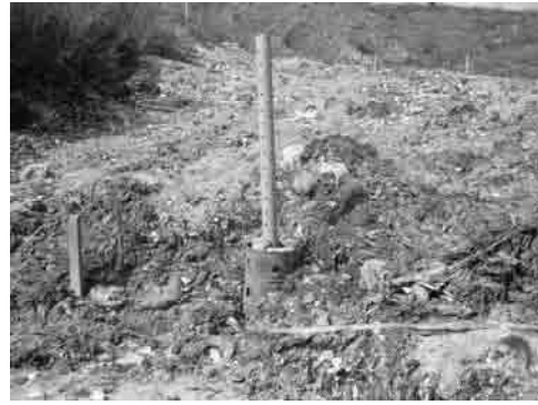
Photo 3.18 Drum Gabion Method
