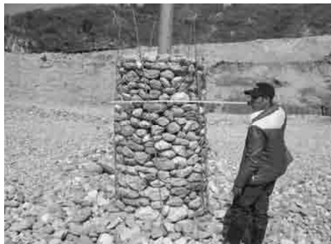
Photo 3.29 Existing Gas Ventilation Facility
