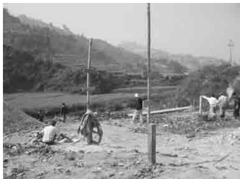
Photo 3.8 Installation of Landfill Height Marker
