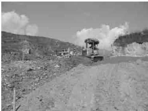
Photo 3.19 Final Soil Cover (No. 1)
