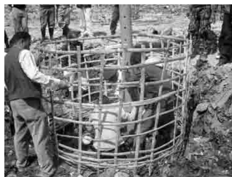
Photo 3.11 PVC Pipe in the Gabion
