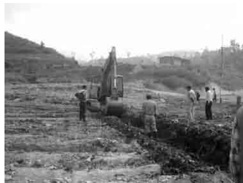
Photo 3.14 Construction of Drainage
