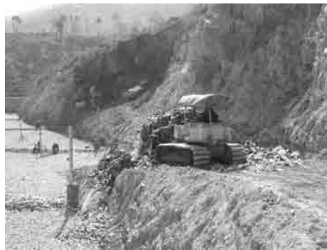
Photo 3.26 Utilization of Bulldozer
