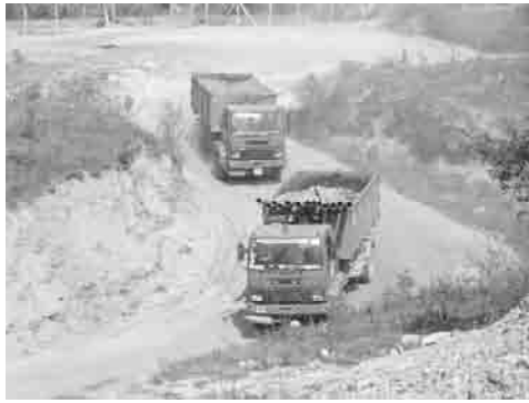
Photo 3.24 Condition of Waste Transportation in Site
