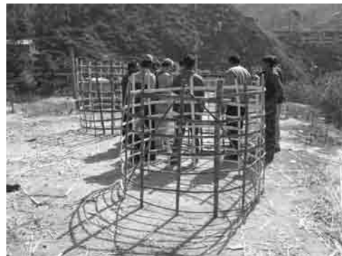
Photo 3.16 Bamboo Gabion Prepared
