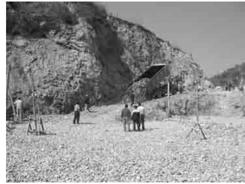
Photo 3.25 Unloading by Dump Truck
