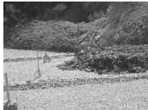
Photo 3.23 Height Markers Installed
