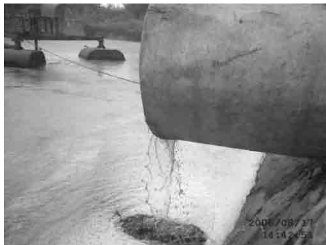
Photo 3 Colored Water Observed at the Exit of Main Collection Pipe
