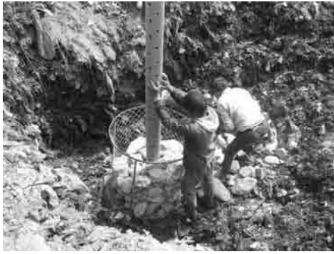
Photo 3.17 Steel Gabion Method
