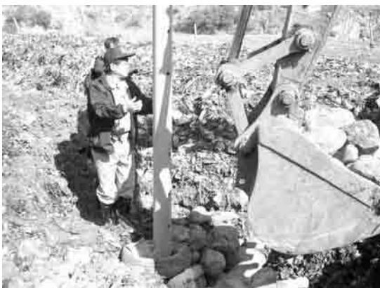
Photo 2.7 Excavation (Before Improvement)
