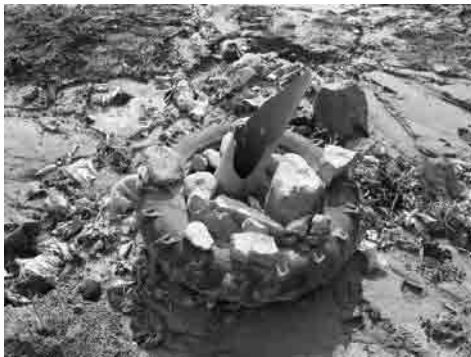
Photo 2.18 Damaged Ventilation Pipe
