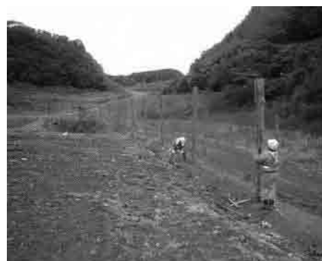
Photo 2.17 Case of Simple Net Installed
