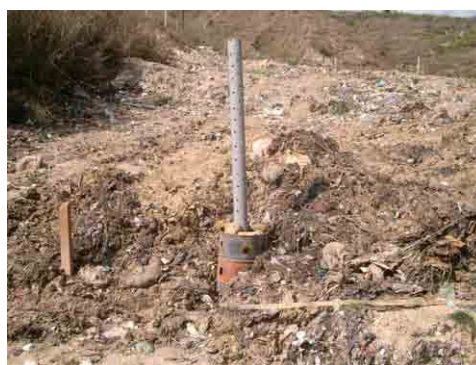
Drum Gabion Method
