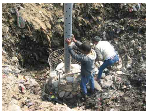
Steel Gabion Method
