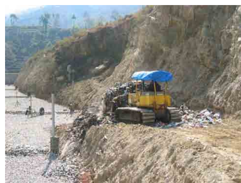
Utilization of Bulldozer
