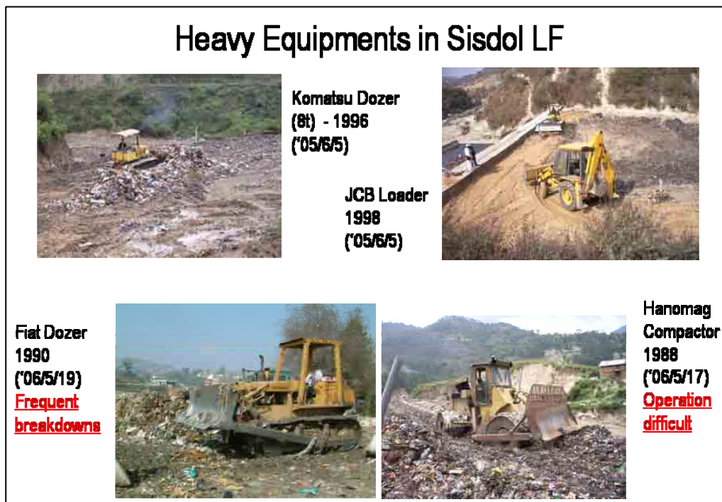
Figure 5.2-3 Heavy Equipments at Sisdol S/T-LF
