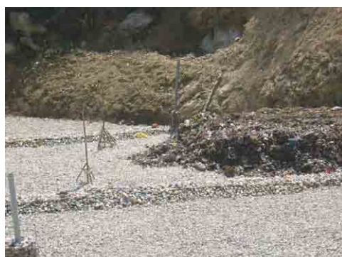
Height Markers Installed
