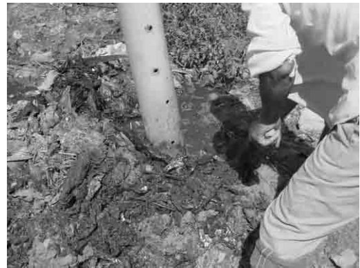
Condition of Gas Ventilation Facility
