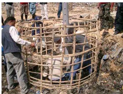
PVC Pipe in Gabion
