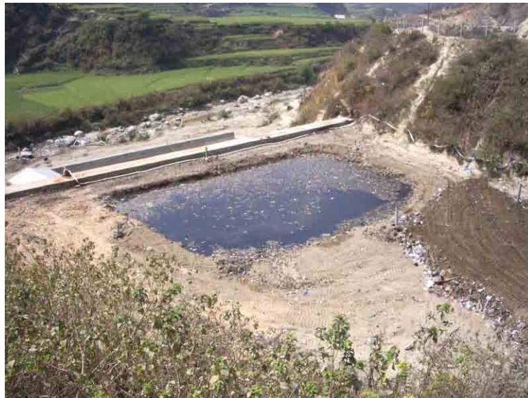
Figure 5.2-7 Photo of Excavated Recirculation Pond (February 2006)
