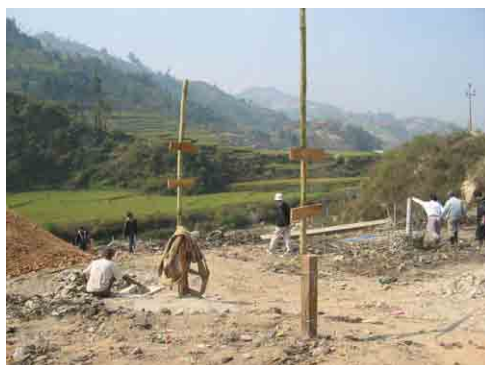
Installation of Landfill Height Markers
