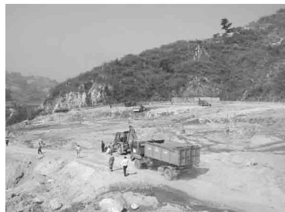
Condition of Sisdol Landfill (March, 2007)
