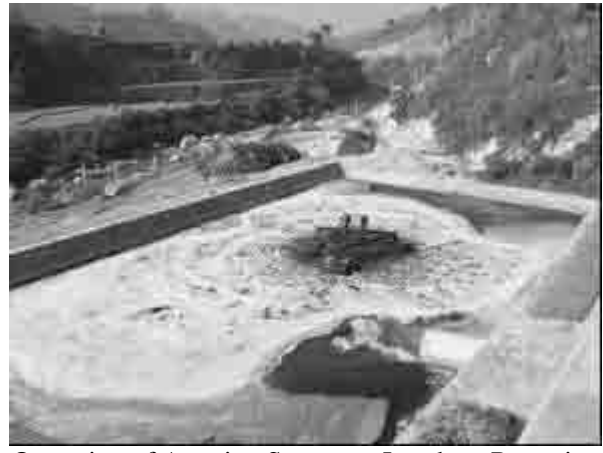
Operation of Aeration System at Leachate Retention Pond (November, 2005)
