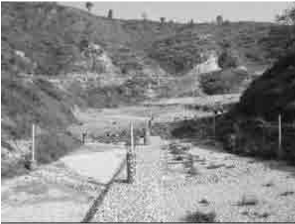
Landfilling Activities at Sisdol Landfill (November, 2005)
