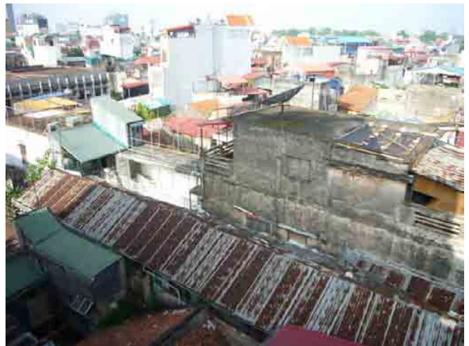
Figure 2.2.4 Inefficient Land Use with Low-Rise Buildings Inside Block
