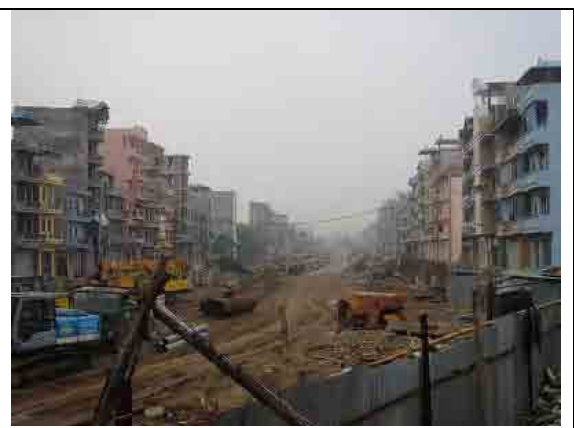
Road expansion projects in the urban center.
