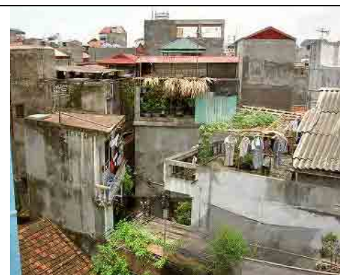
Existing residential area in Dong Da District.
