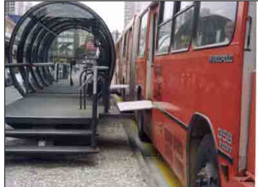
BRT station (Curitiba)
