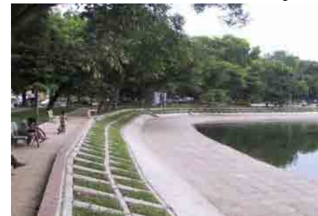
Lake Condition after Restoration (12 July 2005).
