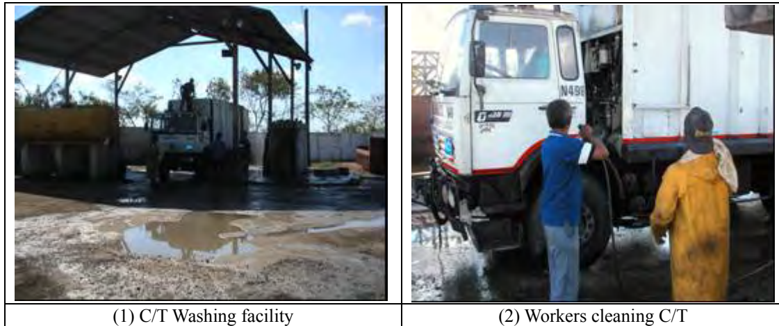
Figure 8 CT Washing Facility
