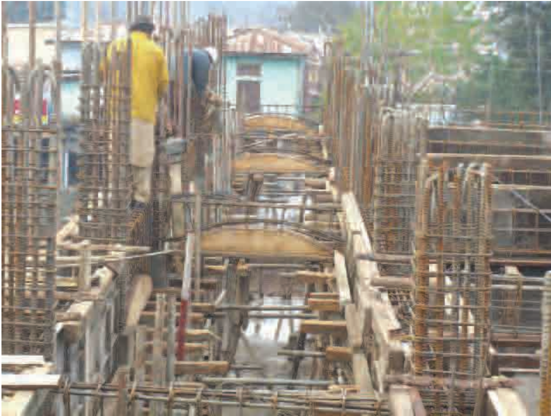
Lower Beam & Column
