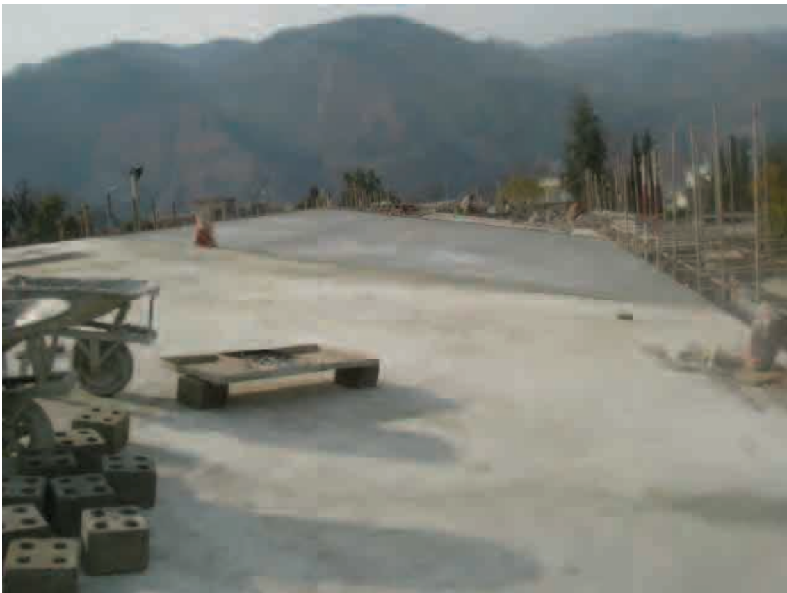
Roof Slab Concrete
