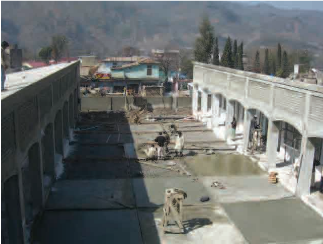
Courtyard Floor Concrete
