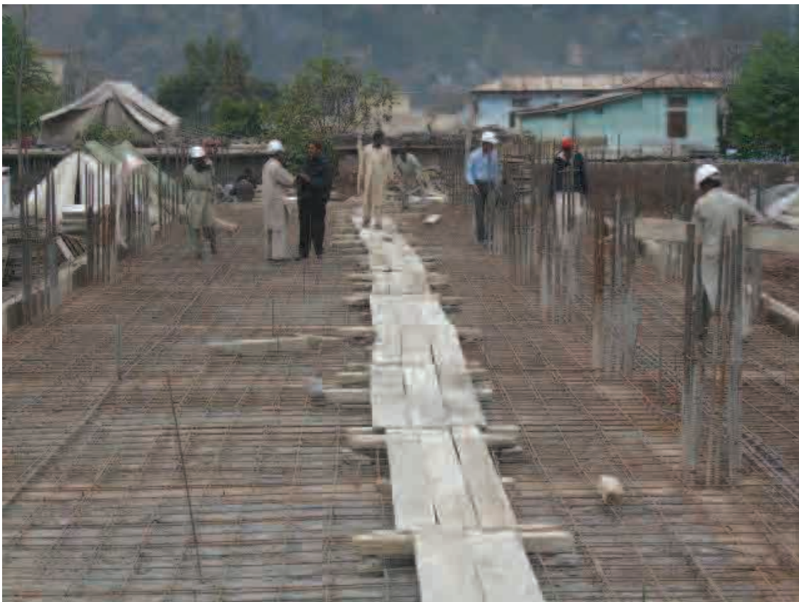
Floor Reinforcement
