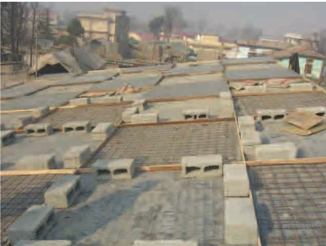
Protect Waterproofing by Mortar
