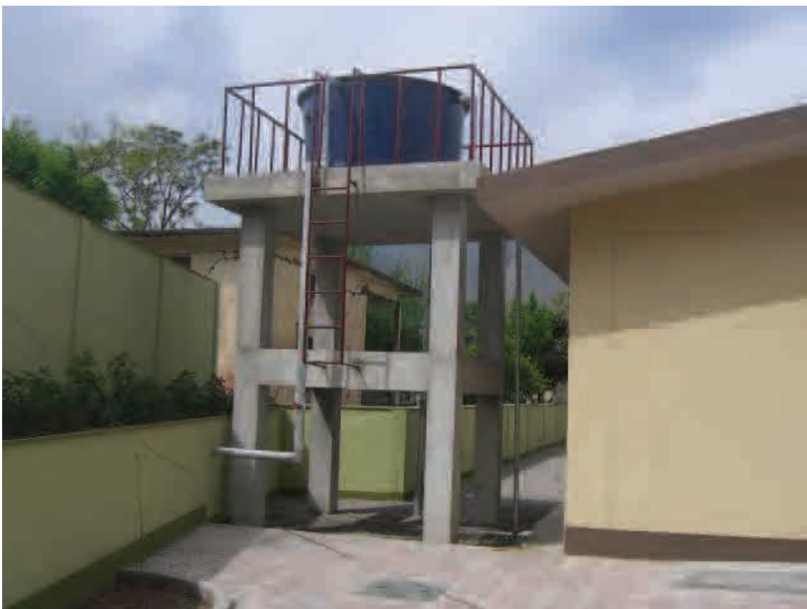
Elevated Water Reservoir
