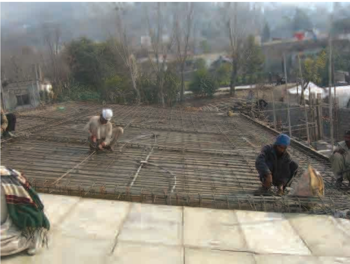
Roof Slab Reinforcement
