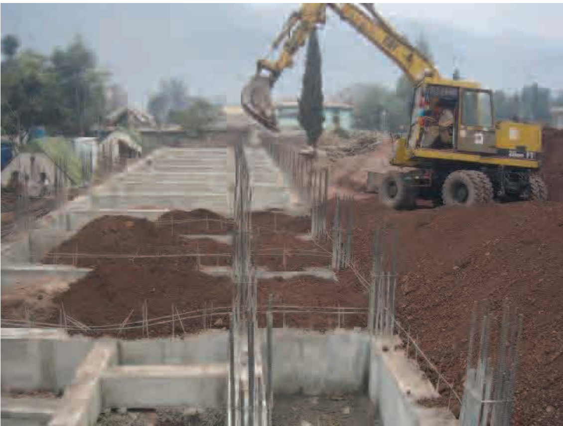
Backfilling
