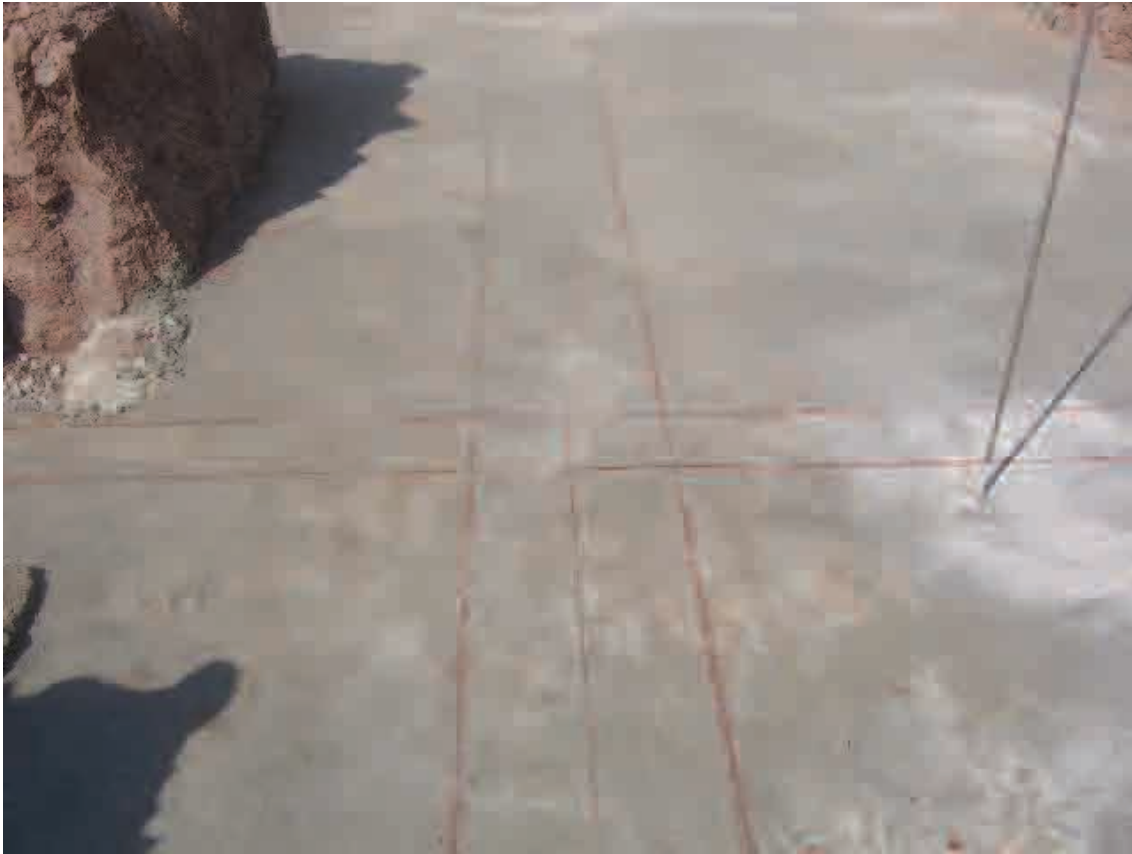
Foundation Beam Marking
