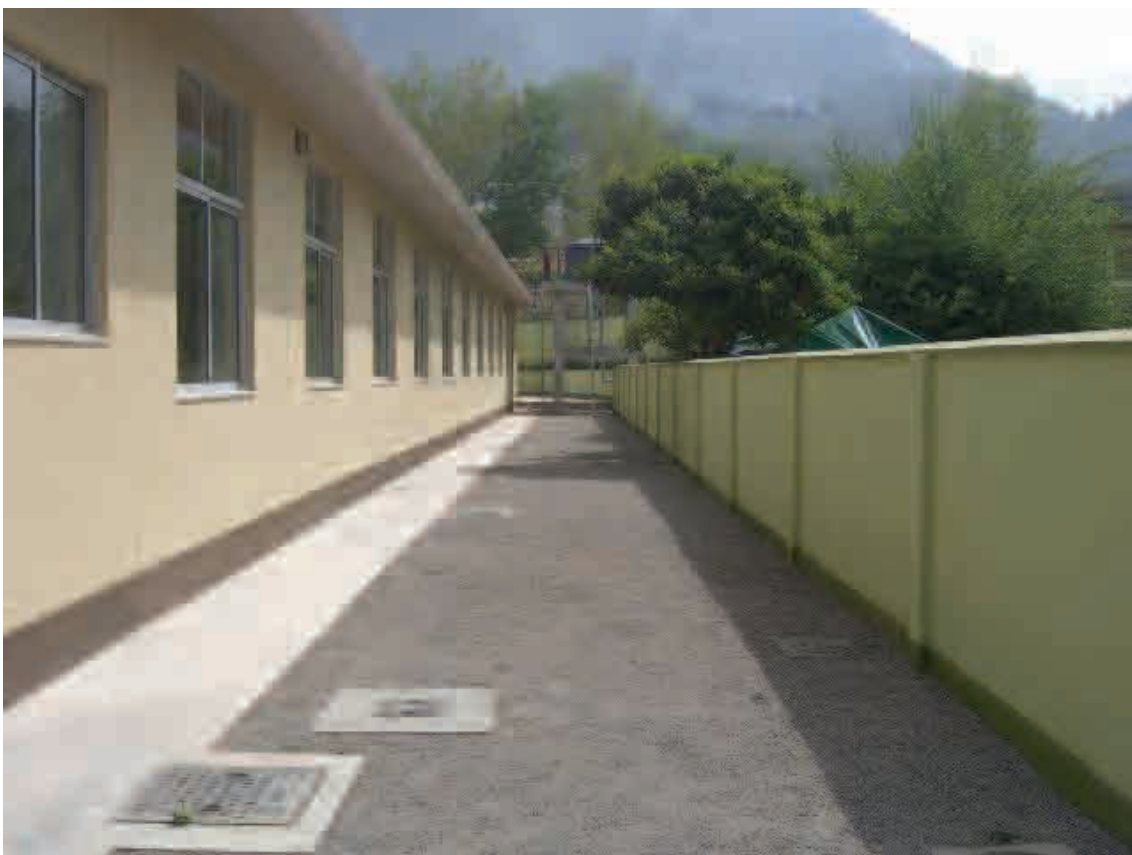
External Wall (South)
