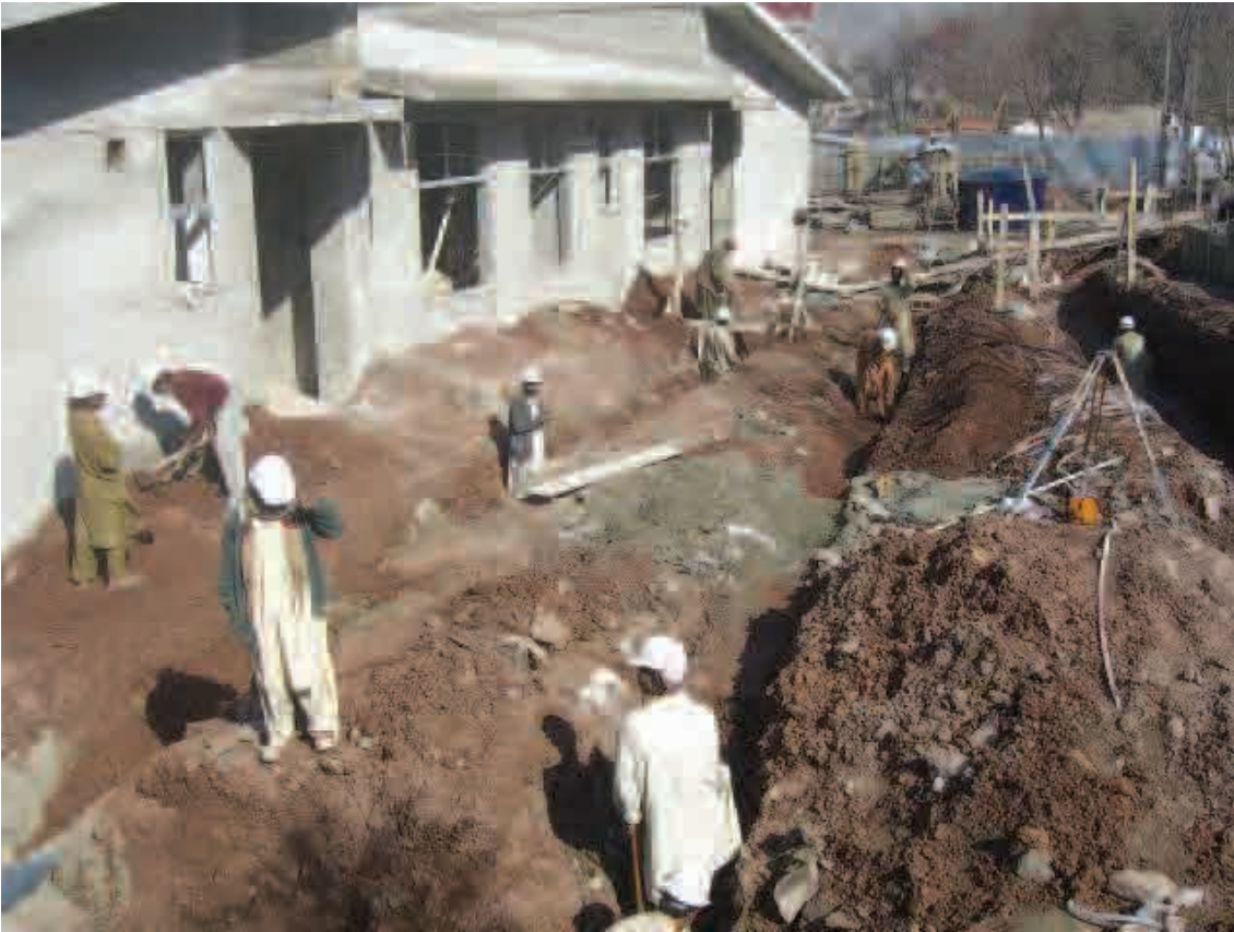
Excavation for Plumbing
