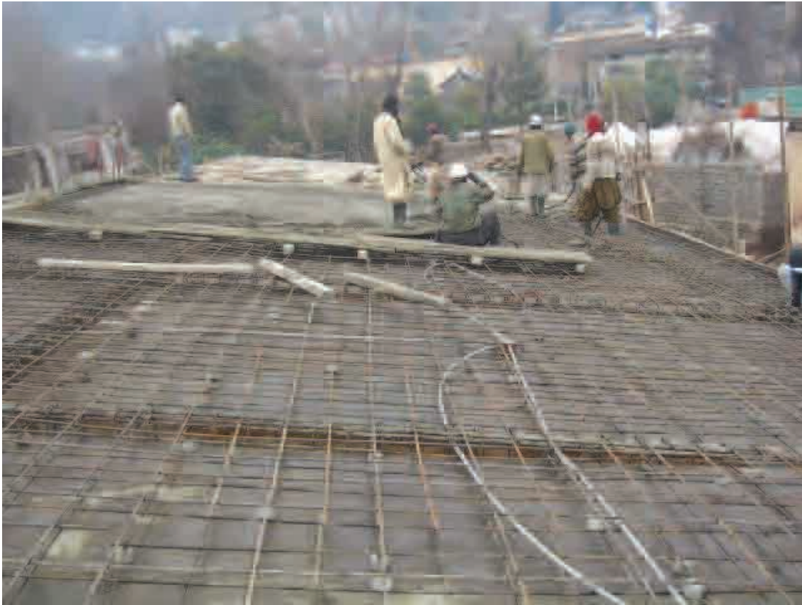
Roof Slab Concrete
