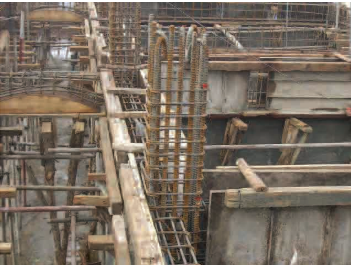
Lower Beam & Column
