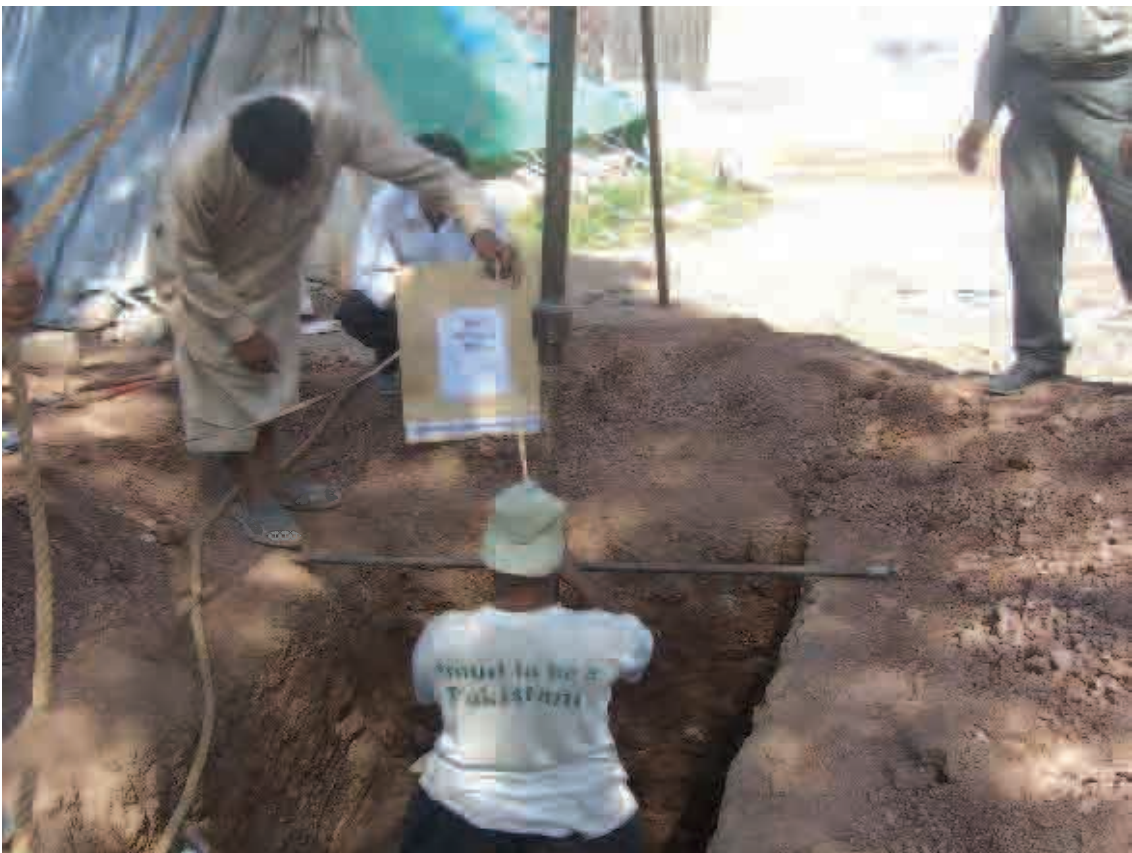
Soil Bearing Test
