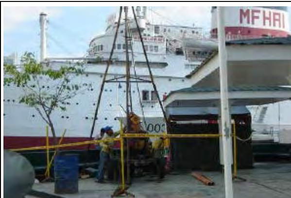
Mechanical Boring at H1CGD
