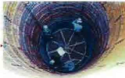
2. Placing liner plate
