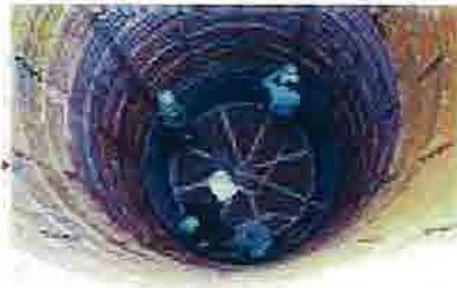
2. Placing liner plate
