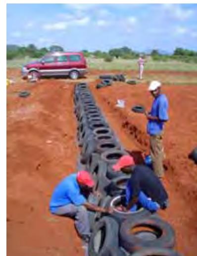
Photo 7.6-4: Constructing aqueduct protection structure with tires in Mankotsana
