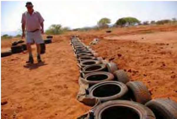
Protection structure with used tires (Community Soil Conservation Project)
