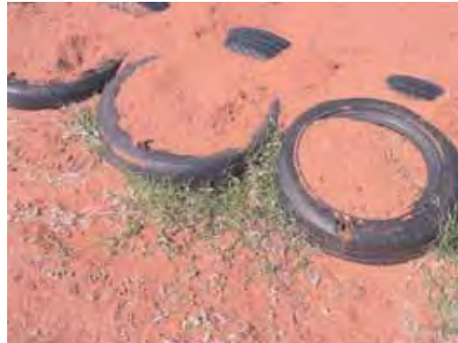
Photo 1 Situation of tire structures just after the flood on 3 March 2006 in Mankotsana - grasses has grown from seeds sown underneath tires, contributing to protection
