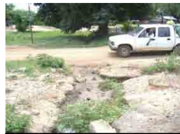
13. Gudele Bridge (new)
